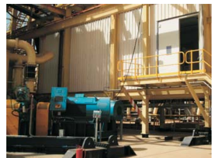
DAKAR, SENEGAL. Installing 14 Siemens Robicon Drives.
